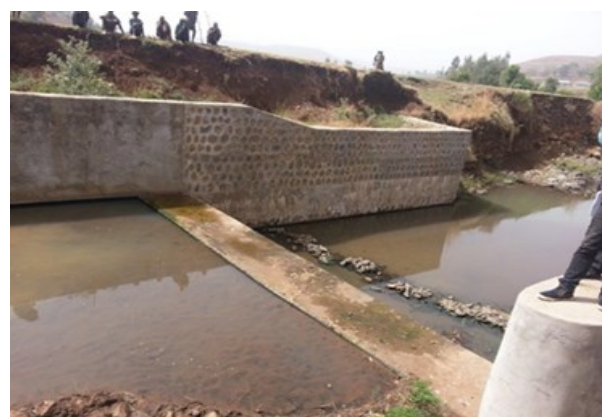
One of the constructed small-scale irrigation schemes
